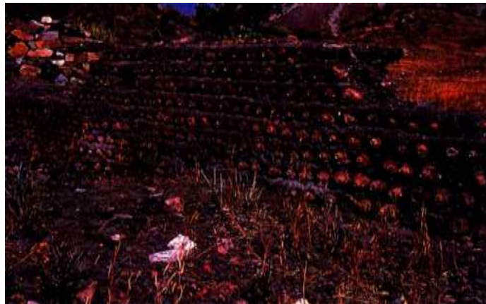
Fig. 3: Residential structures made of discarded retorts
